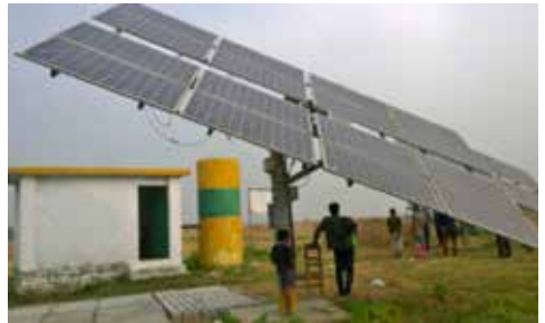
Solar irrigation pumps used for farming in Bangladesh
