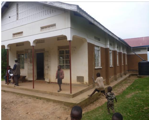
Council hall constructed at Mpungu Sub-County using funds from revenue sharing
