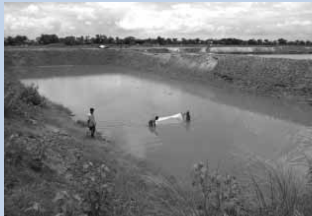
A natural channel of the river is shown which has been modified by earth embankments for use as a closed resource and catchment area for fish culture. The fish including carp will be available nine months of the year. This process involved consensus building over access to the water for the poor. This is a pilot project that ITDG is helping to develop and, if successful, other physical barriers can be more simply erected using netting.
