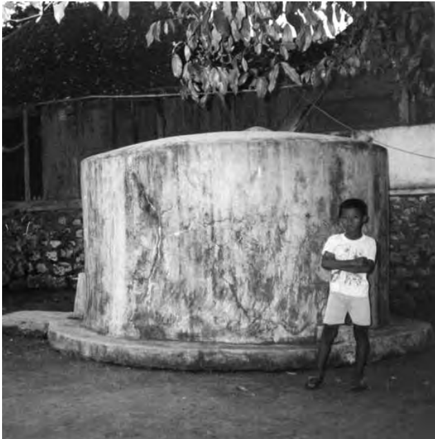
Closed rainwater storage tank
