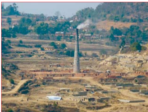
Vertical shaft brick kiln
