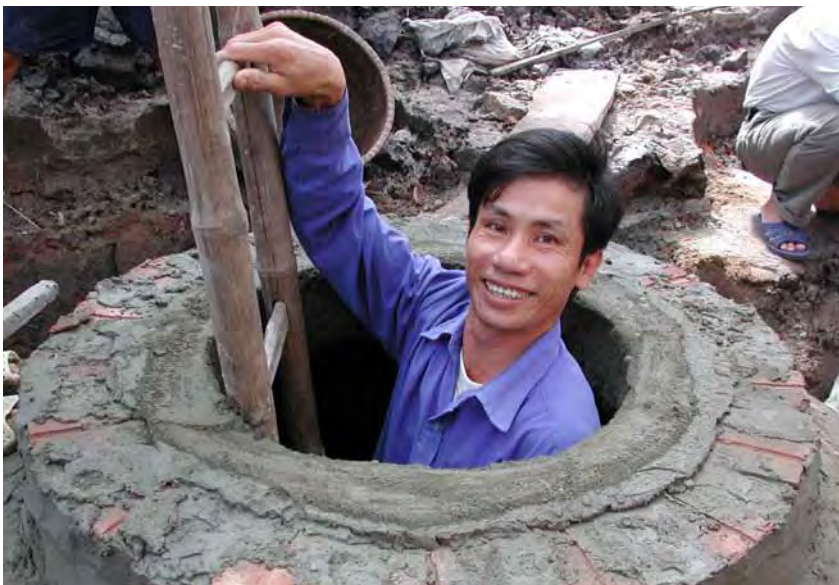
top: Biogas digester, Nepal. bottom: Biogas digester, Vietnam. www.snvworld.org
