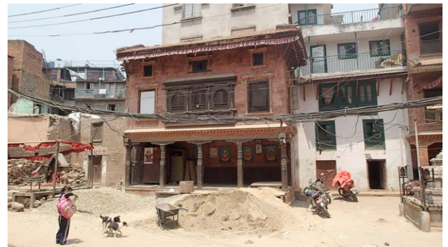
3b: A newly refurbished Newari house in Pilachhen.
