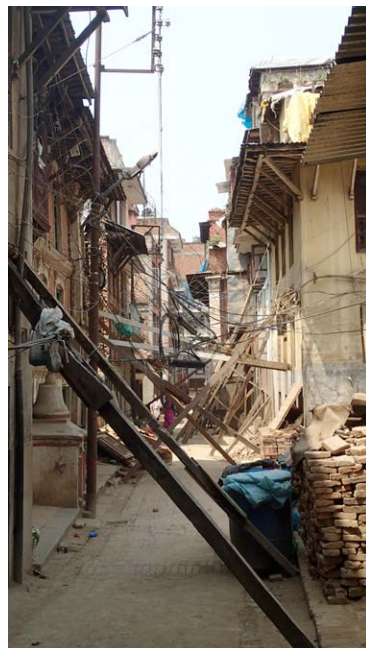
5b: Cross braces in Patan.
