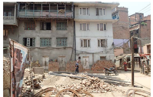
5c: Piles of recycled bricks and building materials in Pilachhen. Photos by Patrick Daly
