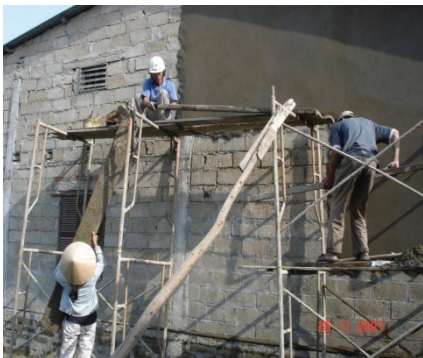
Builders (men and women working together)
