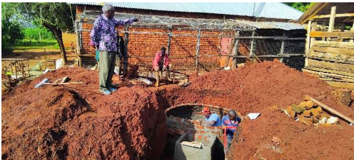
Figure 7. Support from MVIWAMA to install a biogas digester at a member's farm
