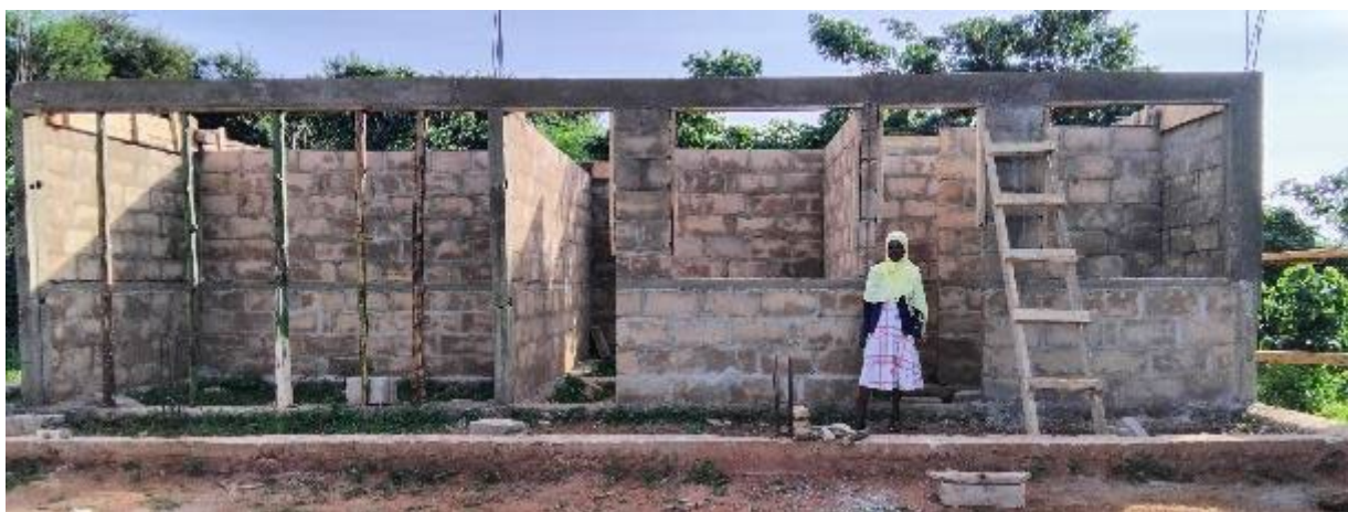
Figure 12. Construction of the Muungano group's honey-processing premises, Bashay village, Mbulu
