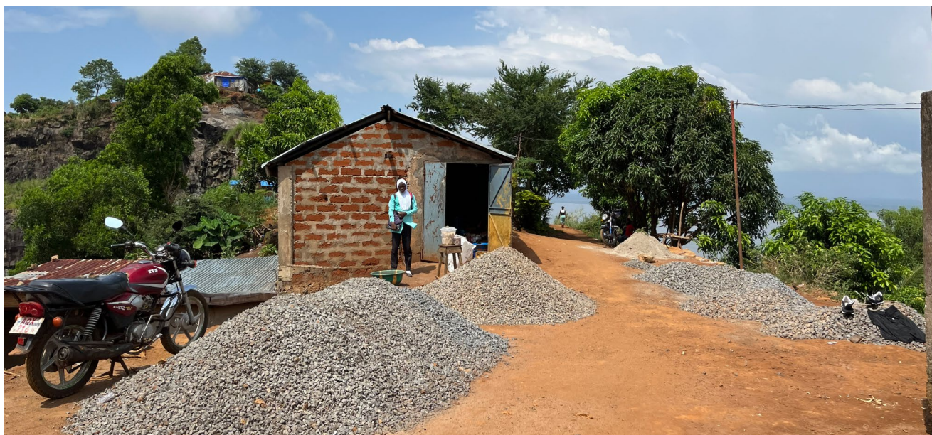
Storage of sand, gravel and rock in Freetown construction site. Credit: Camila Cociña/IIED
