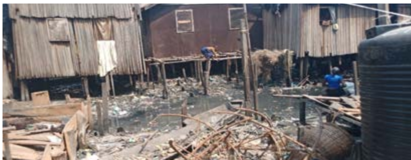
Figure 4. A black water tank, with no power source to pump in clean water. The community lacks access to clean water for drinking and other necessities. Damaged buildings lead owners to explore coping measures, such as using waste to reduce the flow of water. Such measures prevent future flooding incidents from causing further damage. Credit: Samuel C. Okorie
