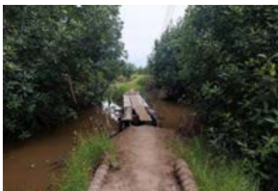
Figure 11. A footpath and an artisanal bridge, linking Havui and Adidokpo, with mangrove forests on each side. Also at the sides are coconut stems placed to reduce the erosion of sand from the footpath. Credit: Sylvanus S.P. Doe
