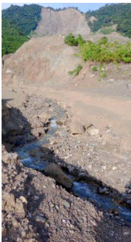
Figure 5. Multiple landslides have destroyed buildings and land crucial to the community's subsistence lifestyle. Credit: Santo Sunset Environment Network
