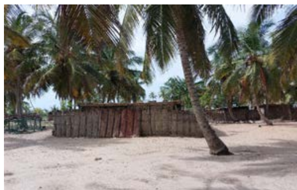
Figure 13. Some residential buildings are eco-friendly and cost-effective but they cannot withstand climate extremes, necessitating a new eco-design for infrastructural development at Fuveme. Credit: Sylvanus S.P. Doe
