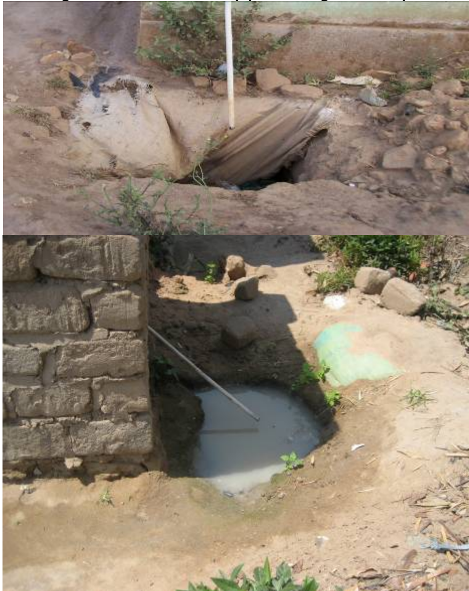
Figure 9a: Urine-diversion pipes leading into soak pits
