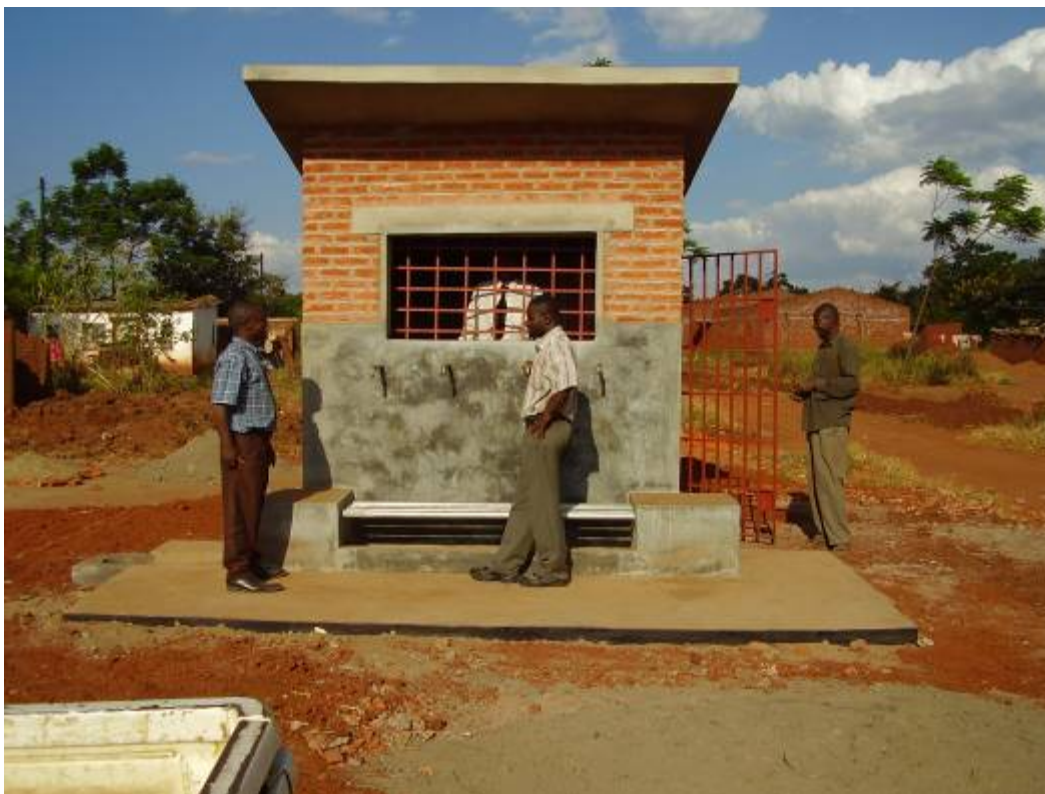
Figure 6: Newly built water kiosk in Area 24, Lilongwe; the cost of the kiosk is reflected in the cost of water
